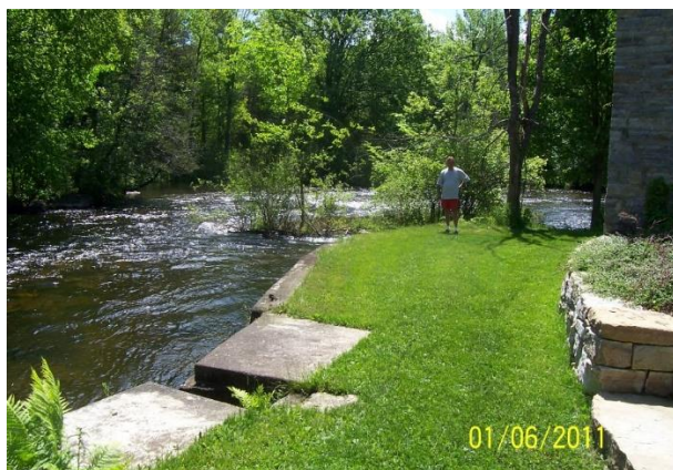
Mill Shore Foundation & Sluice Area
