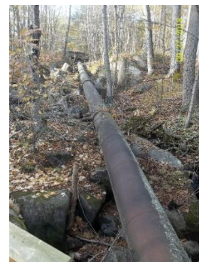
Pipe from dam to Mill
