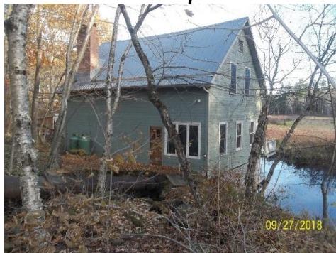
Rear View of Fream Mill
