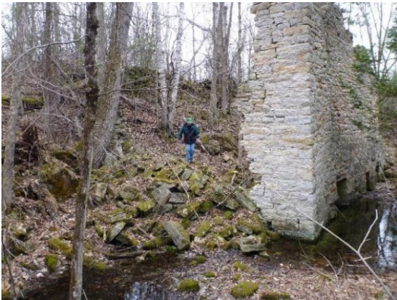
Downstream Side of Woolen Mill With Water Conduits at Base
