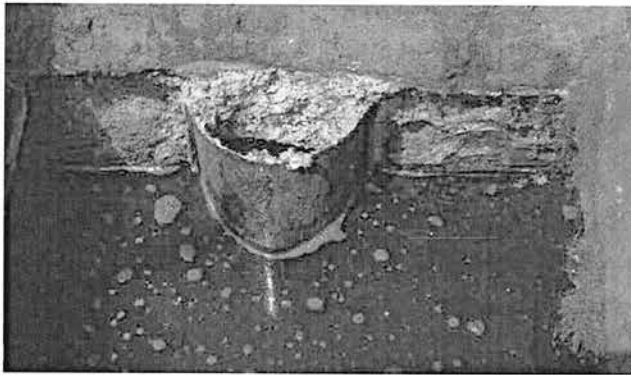
Photo 1: Concrete Corrosion around Outlet Baffle
