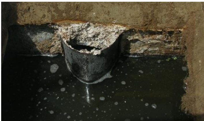
Photo 1: Concrete Corrosion around Outlet Baffle
