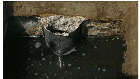
*Illustration 1: Concrete Corrosion
