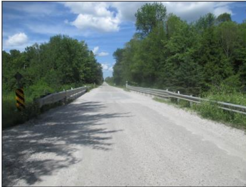
Roadway looking East.
