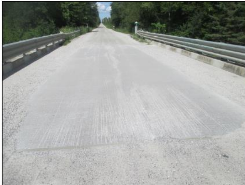
Deck top showing abrasions.
