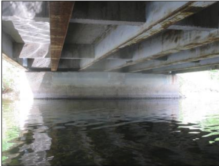
East abutment, showing scaling at waterline (typ.)
