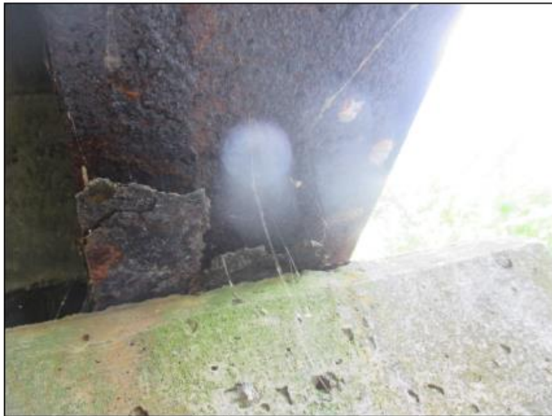
Corrosion and medium section loss at girder end (typ.)
