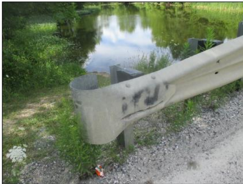
Damage at North-West guiderail.
