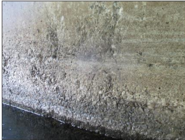
Severe scaling at waterline on abutments.
