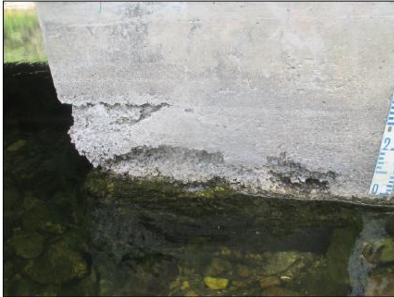
Very severe honeycombing of North-West wingwall.
