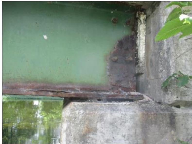
Section loss at girder end.
