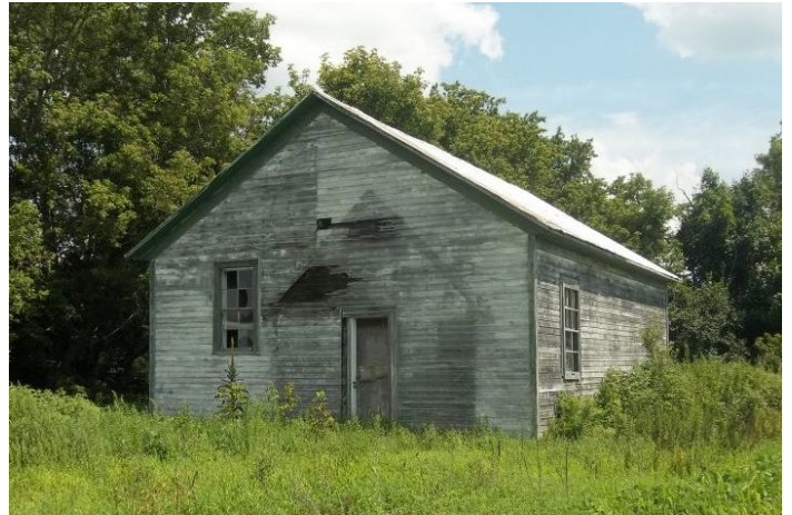
S. S. # 7 building – in 2016 (D. Taylor photo)
