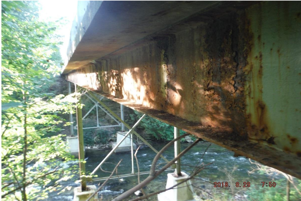
Photo 9: East Exterior Girder – Light to Medium Corrosion
