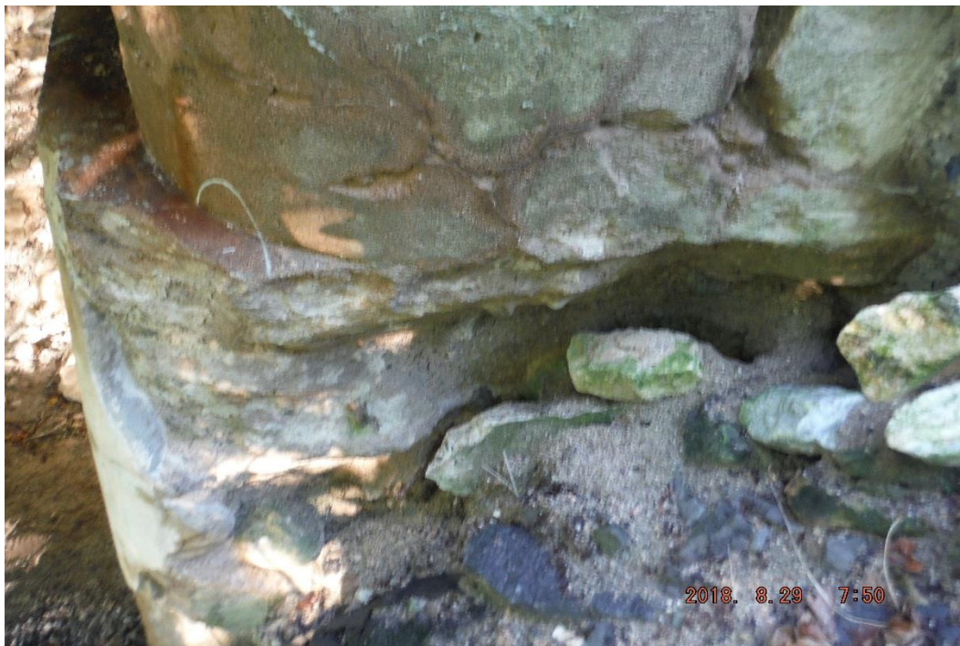
Photo 23: Northeast Wingwall – Severe Erosion, Scaling and Disintegration
