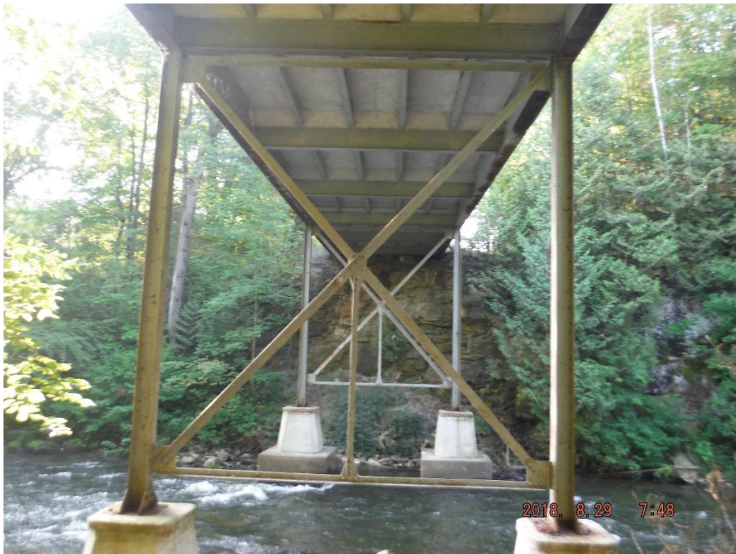
Photo 16: South Pier System – Light to Medium Corrosion
