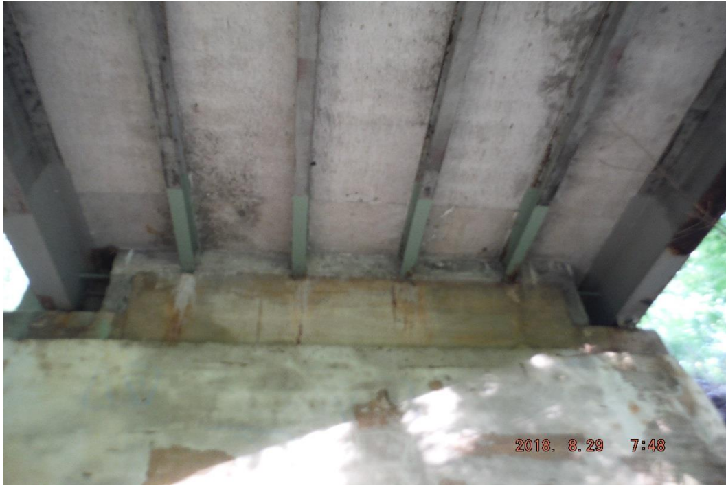
Photo 15: North Beam Ends, Ballast Wall and Stringers
