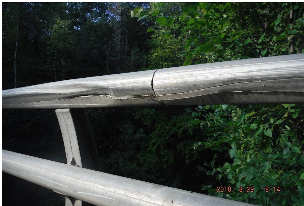
Photo 4: East Railing System – Collision Damage
