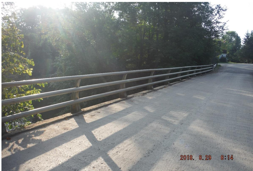
Photo 3: West Railing System
