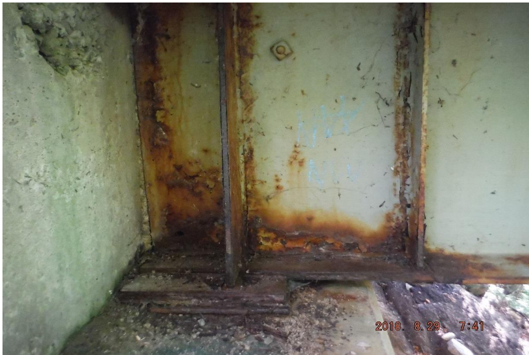
Photo 10: Northwest Girder End and Steel Bearing – Light to Medium Corrosion
