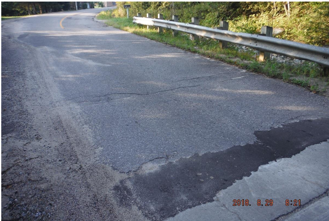
Photo 2: South Approach – Medium to Severe Cracking, Light to Medium Raveling and Asphalt Patch
