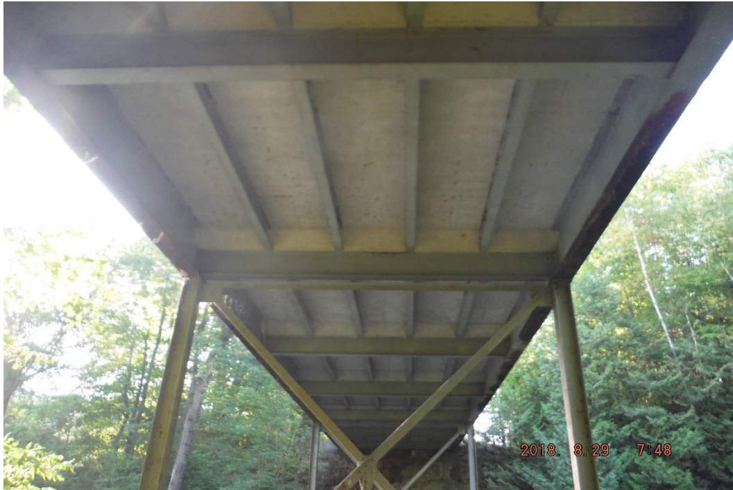
Photo 13: Interior Soffit, Stringers and Floor Beams
