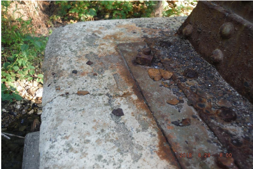
Photo 19: Northeast Pier Pedestal and Bent Connection – Wide Crack and Medium to Severe Corrosion
