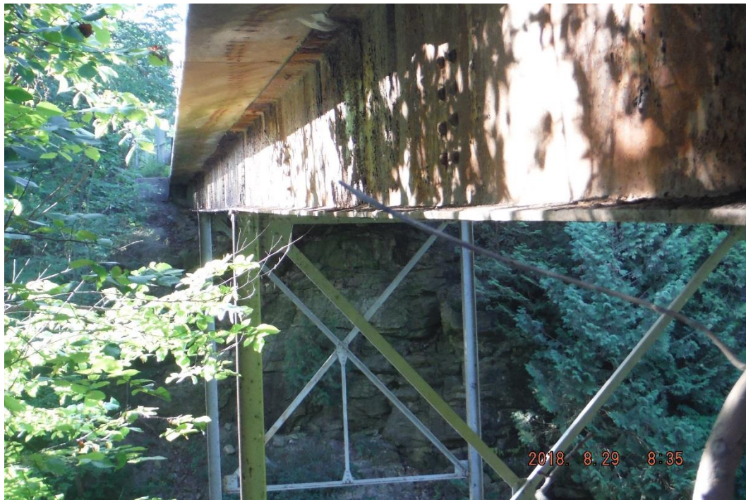
Photo 14: East Exterior Soffit – Light Delaminations and Hairline to Narrow Cracking
