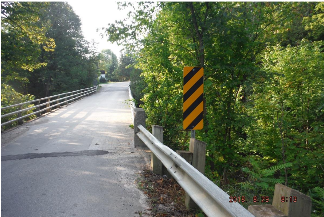
Photo 6: Southeast Hazard Sign
