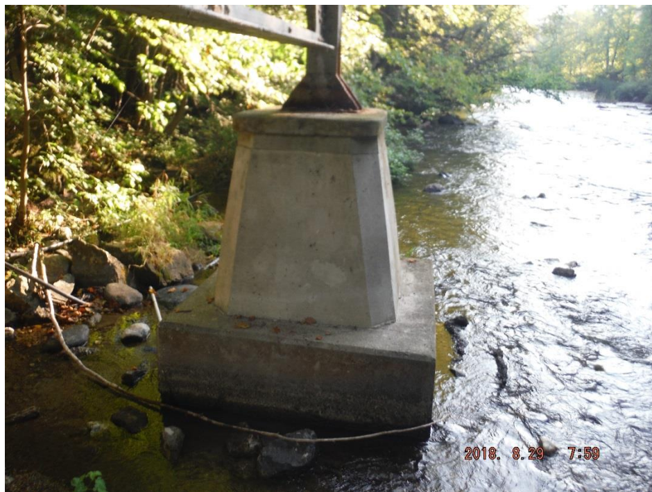
Photo 18: Northeast Pier Footing and Pedestal – Light to Medium Scaling and Medium to Wide Cracking
