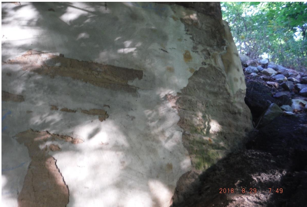
Photo 21: North Abutment on the East End – Severe Delaminations and Severe Erosion and Disintegration
