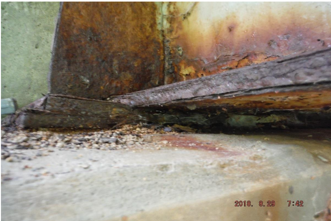
Photo 12: Northwest Bearings – Medium Corrosion and Deformations
