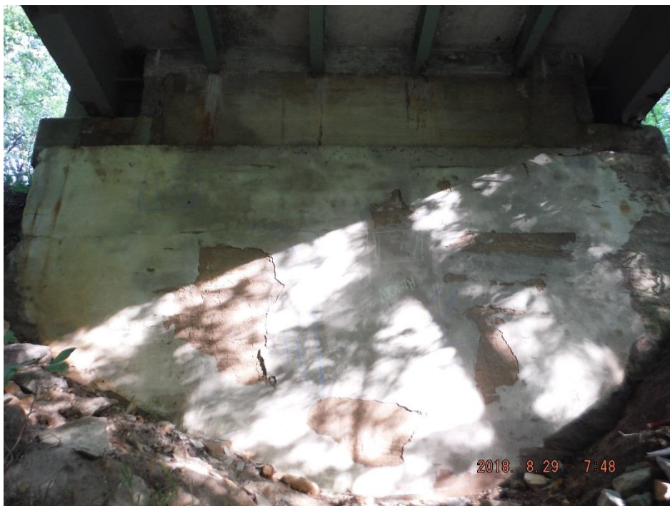
Photo 20: North Abutment Wall – Severe Delaminations, Wide Cracking, Severe Scaling and Disintegration
