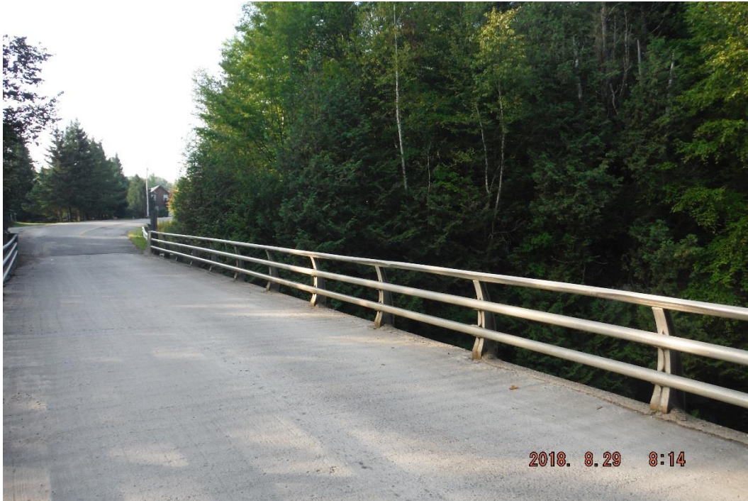
Photo 7: Exposed Concrete Wearing Surface
