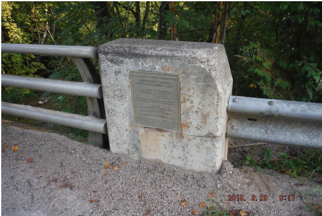
Photo 5: Northwest Concrete End-Post – Medium Scaling, Light Spalling and Light Abrasions
