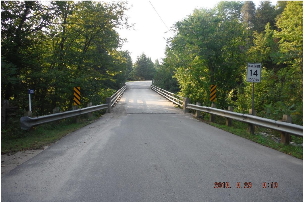
Photo 1: North Approach Looking at Structure
