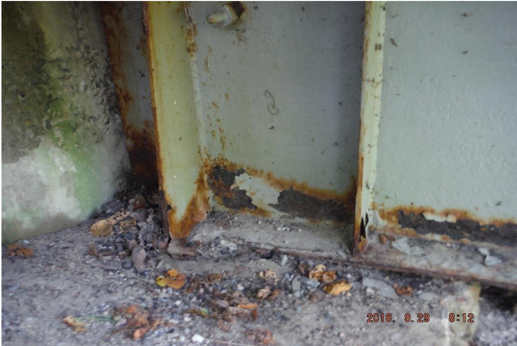
Photo 11: Southeast Girder End – Light Corrosion and Excessive Debris on Bearing Seat
