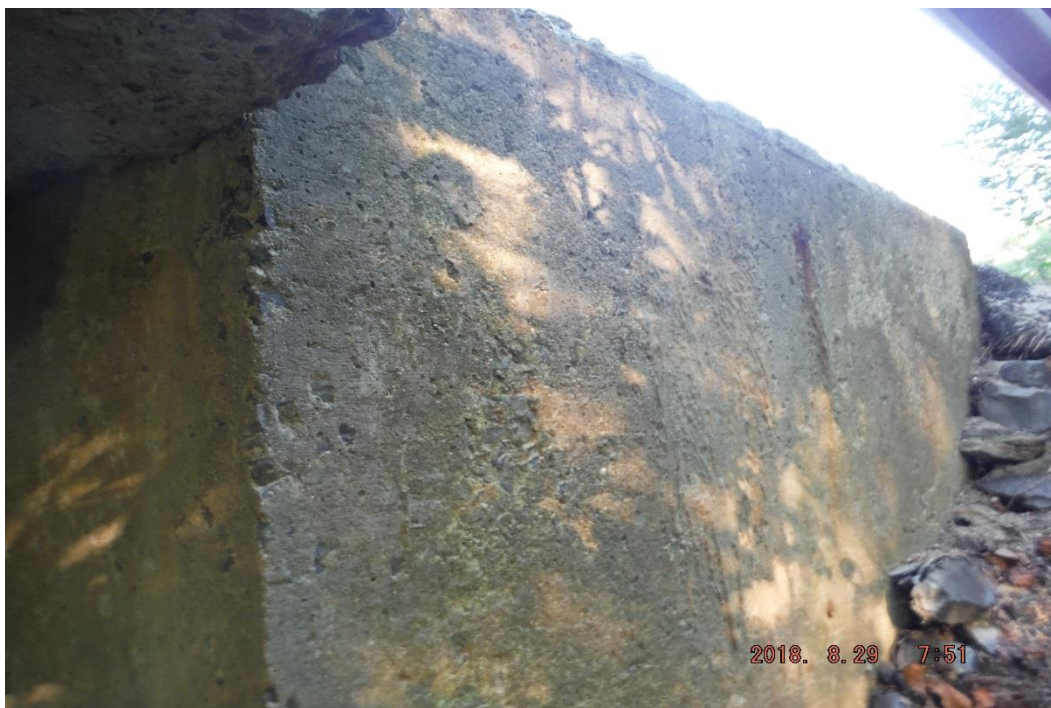
Photo 22: Southwest Wingwall – Light to Medium Scaling
