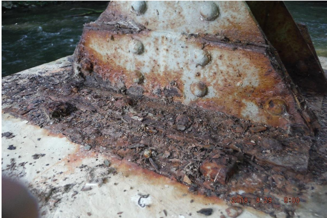
Photo 17: Northwest Pile Bent Connection – Severe Corrosion with Section Loss
