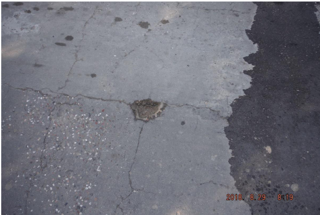
Photo 8: North End of Deck – Severe Delaminations, Light Spalling and Medium to Wide Cracking
