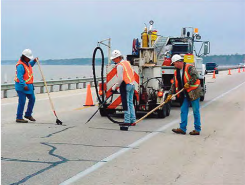
Crack Sealing
