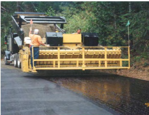
Surface Treatment (Chip Seal)
