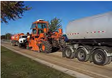
Expanded Asphalt Stabilization
