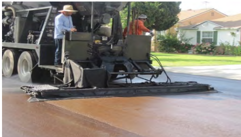
Slurry Seal
