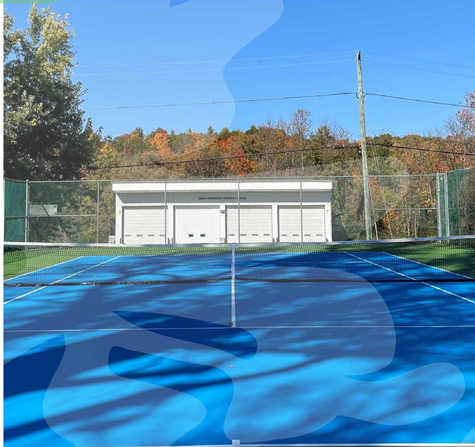
Newly resurfaced tennis court at Maberly
