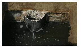
Illustration 1: Concrete Corrosion around Outlet Baffle
