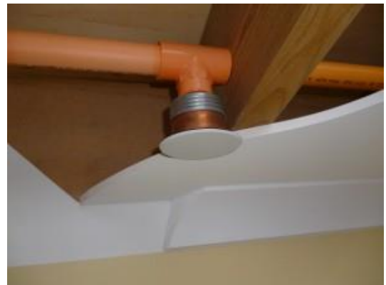
Figure 18: Example of a Concealed Residential Fire Sprinkler
